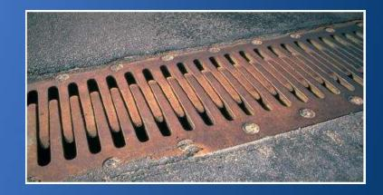
Joints such as this one are used in bridges to accommodate thermal expansion.
